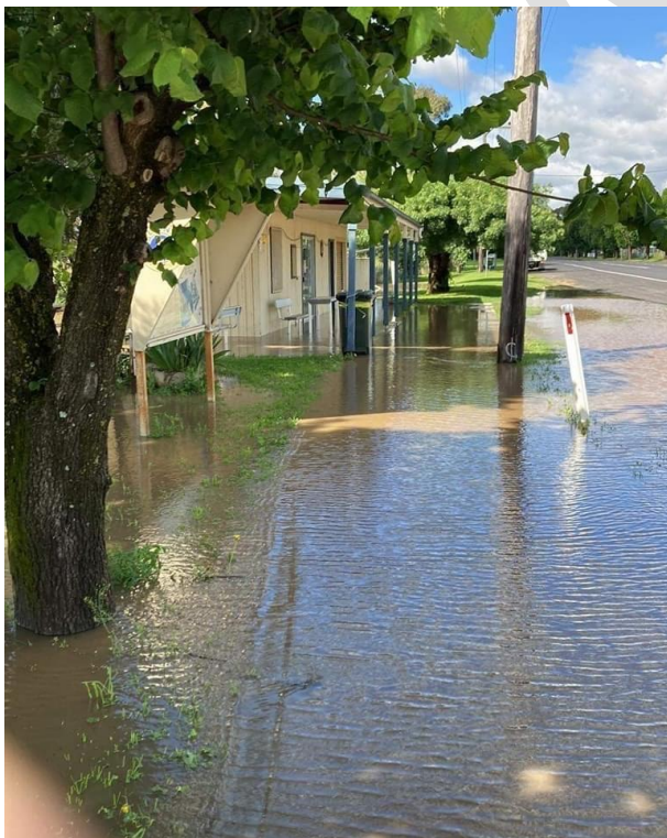
Image 13: Public submission of flooding event at Binnia St near building
