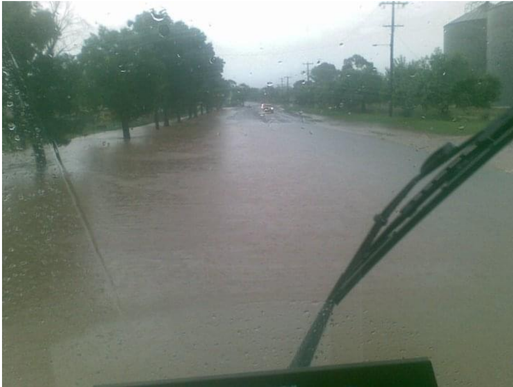
Image 12: Public submission of flooding event at Binnia St near grain silos
