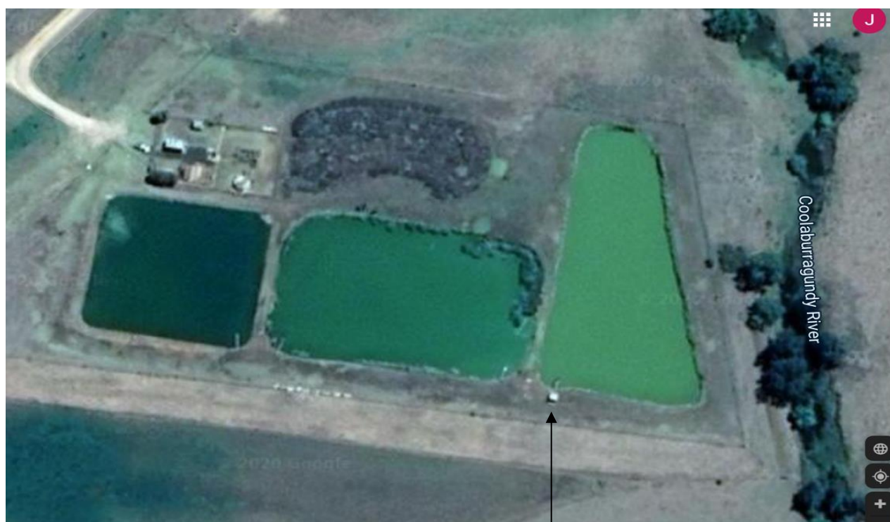
Decommissioned pit and pipeline
