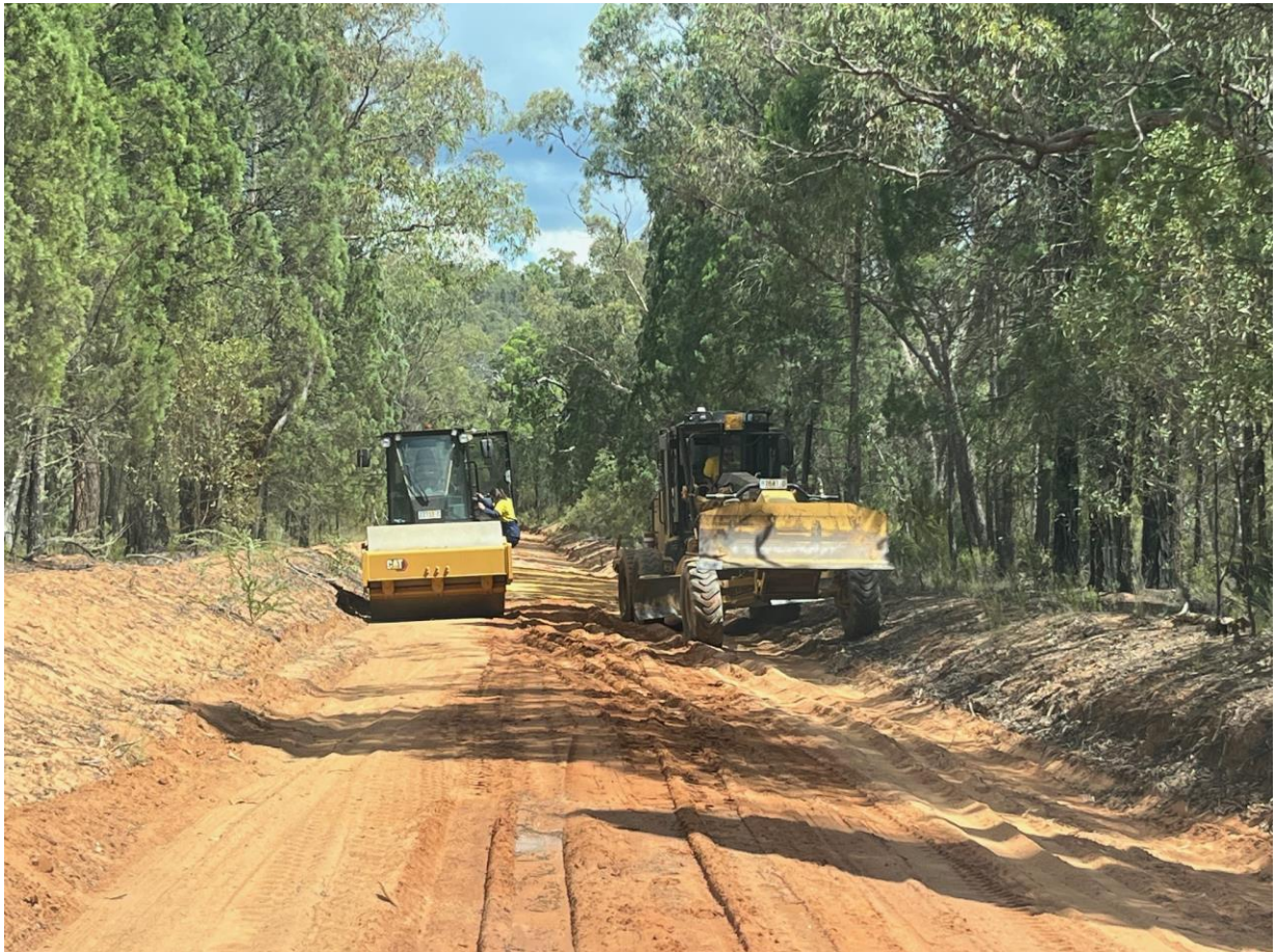
Photo: Road Crews working on Tothills Road, Coonabarabran.
