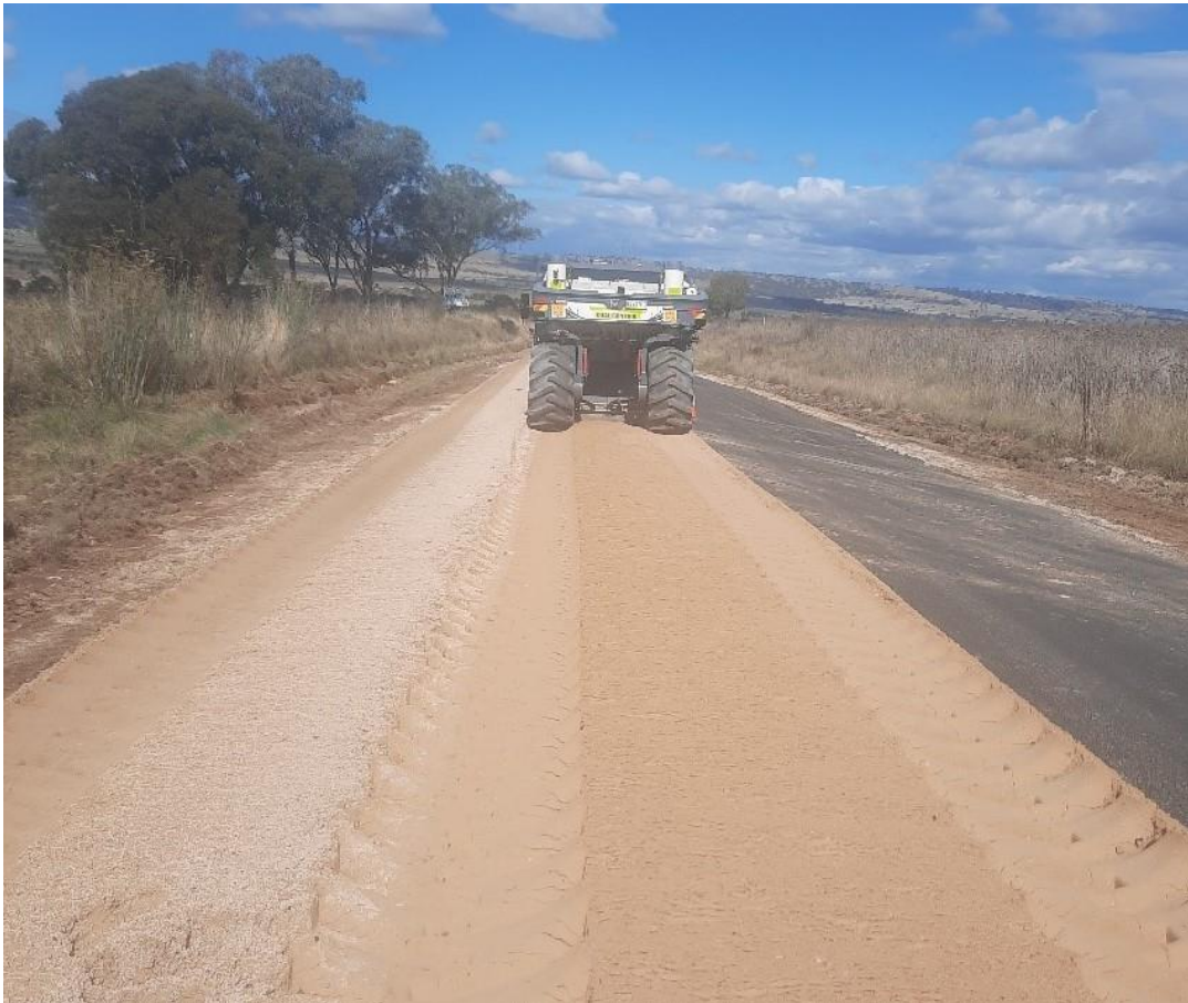
Photo: Works underway on Black Stump Way near Coolah
