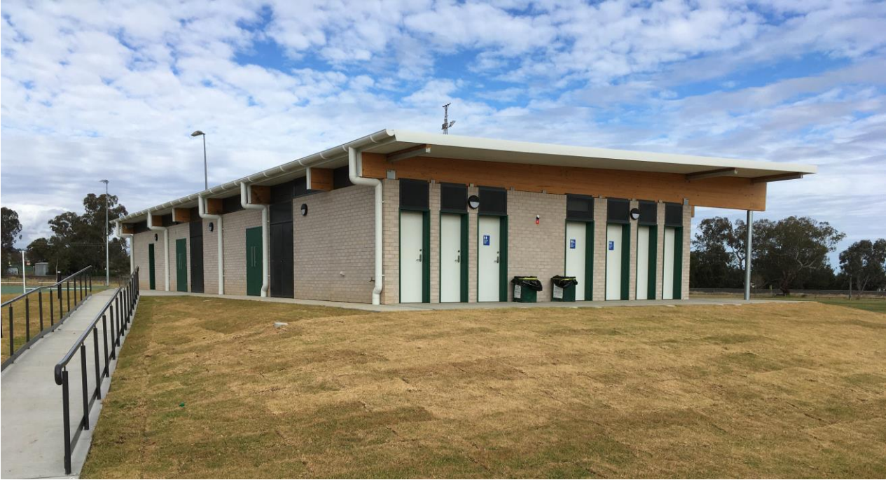
Photo: New Robertson Oval Amenities Building
