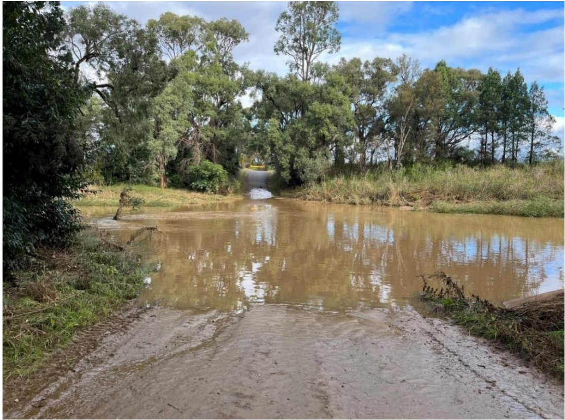
Photo: Merrygoen Creek Causeway on Yarrow Road, Mendooran
