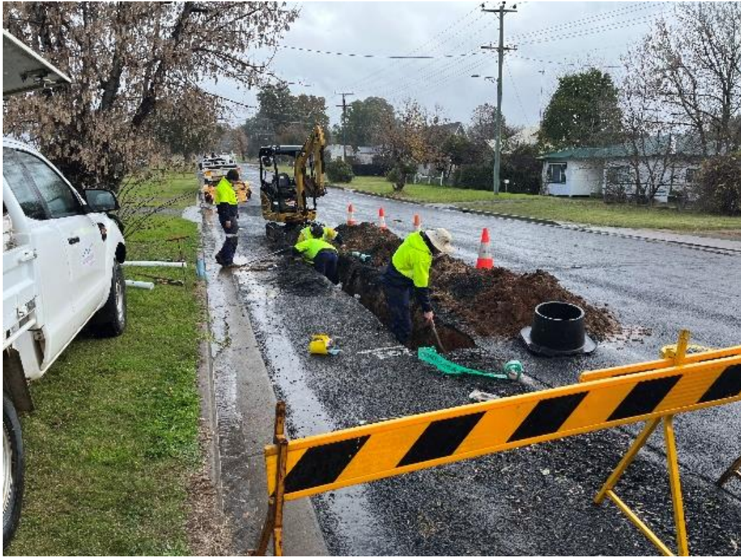
Pictured Above – Council crews working on the Cassilis St project
