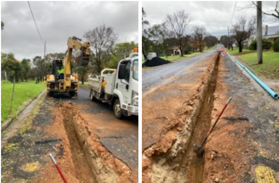
Pictured Above – work on Scully Street project, Coolah
