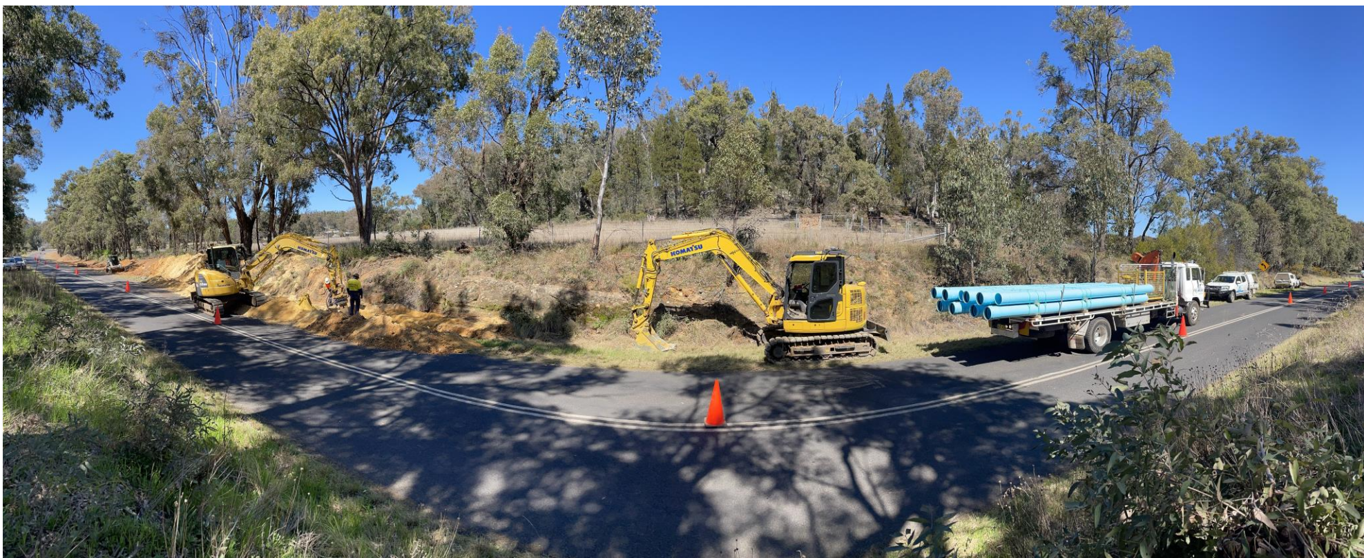
Photo: Working being undertaken along Timor Road, Coonabarabran.
