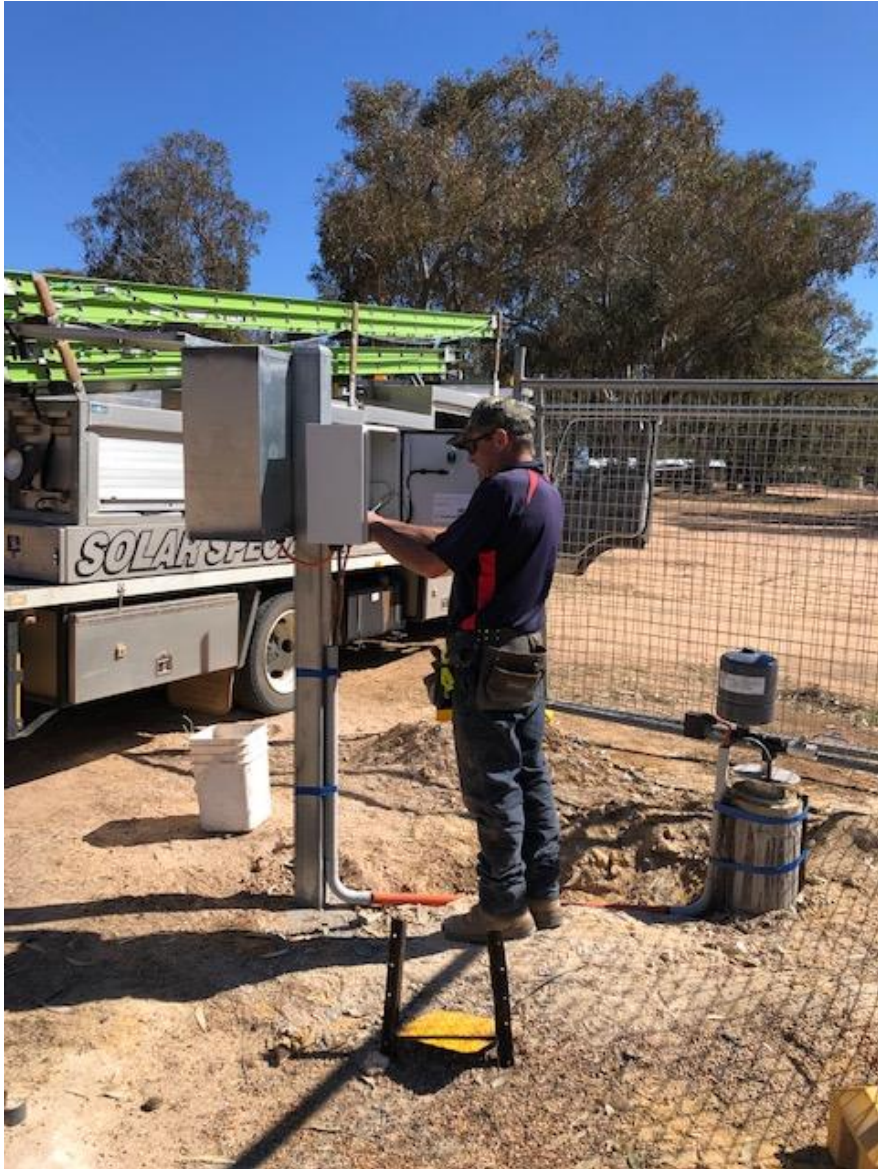
Image: Finalising the finishing touches of the Bore.
