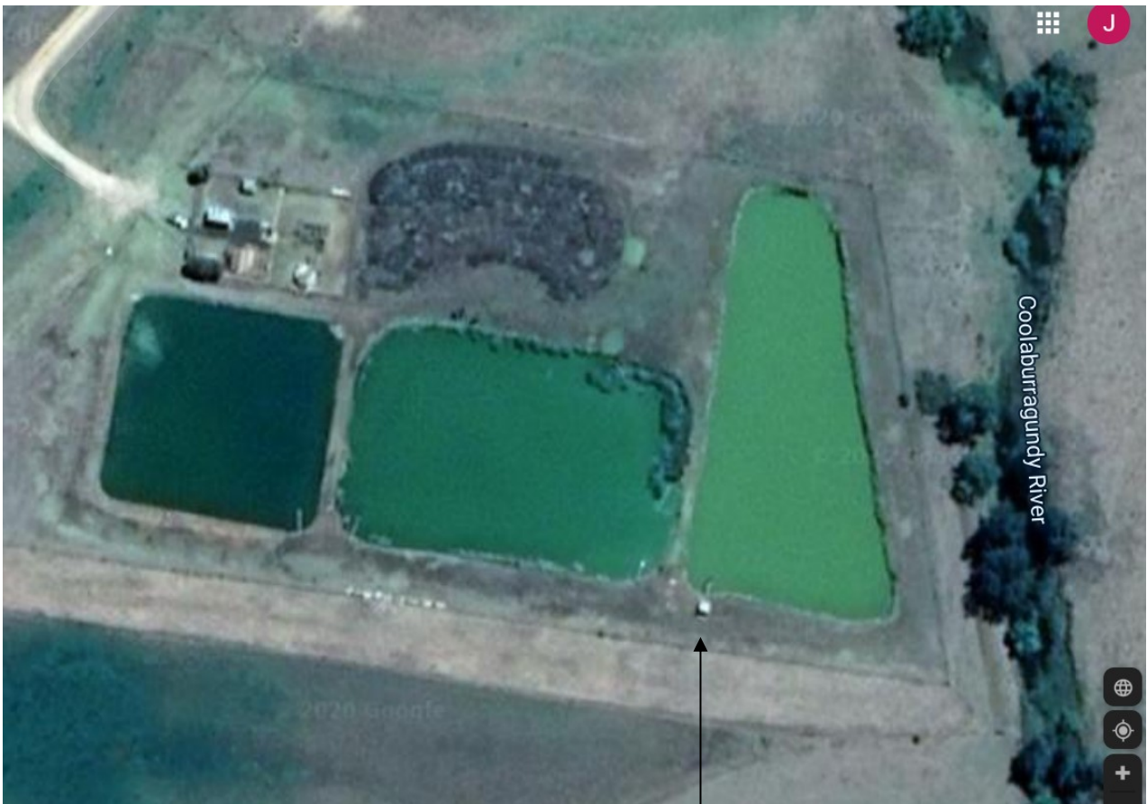
Decommissioned pit and pipeline
