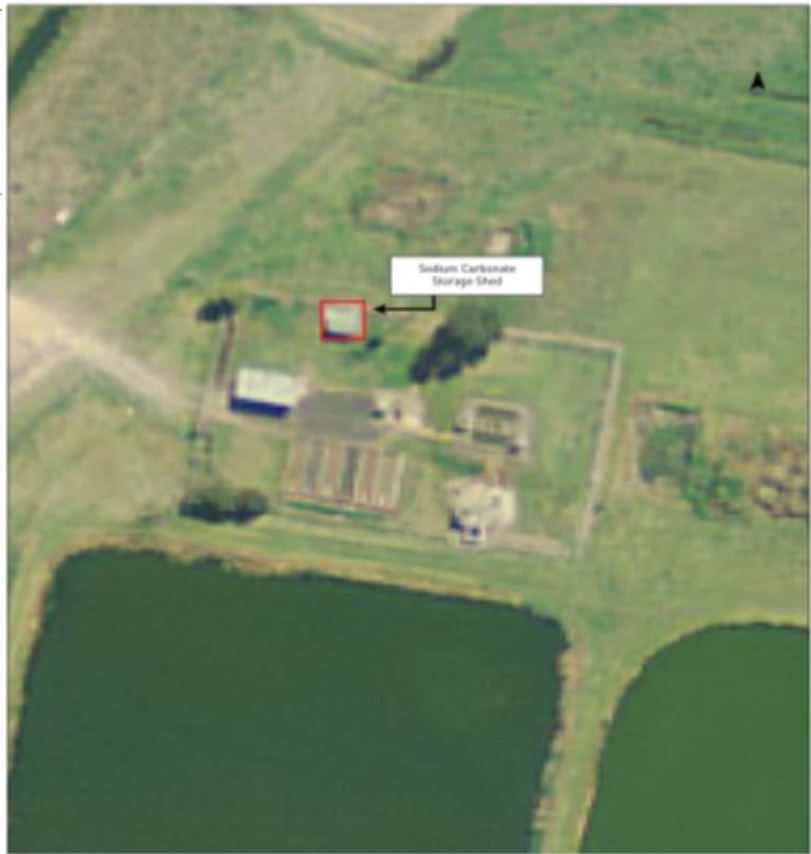
Coolah Sewerage Treatment Plant
