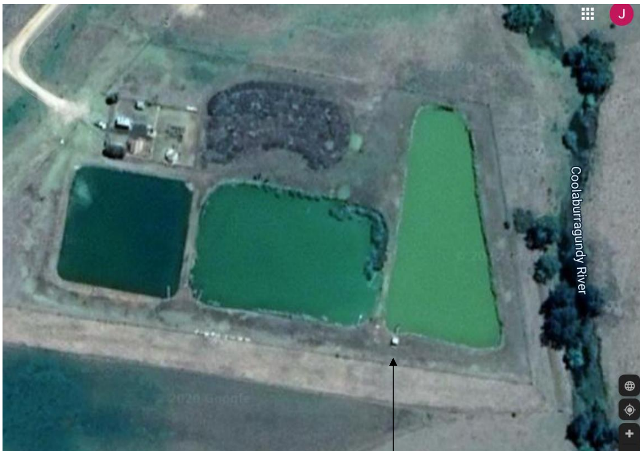
Decommissioned pit and pipeline
