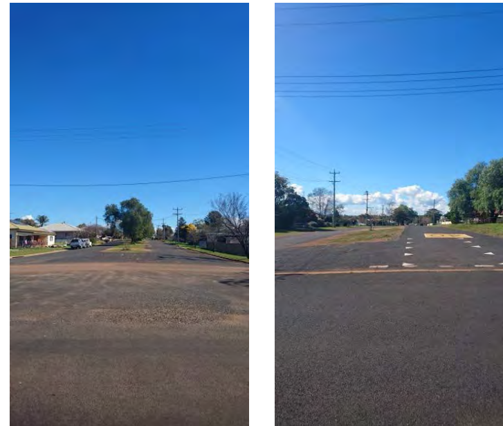
Figure 2. Existing conditions. Left image: Western end of Cobbora Street, near the Pre-School. Right image: Eastern end of Cobbora Street, near the Sports Club.
