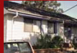
Cladding hiding fibro walls
