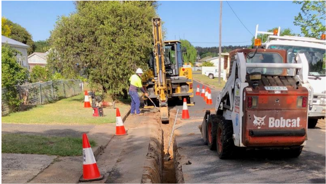
Photo: King Street Water Main Replacement
