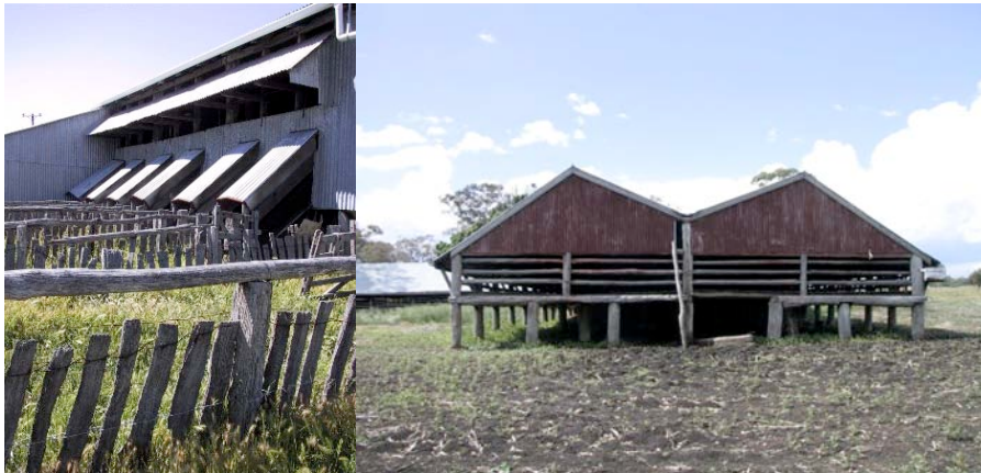
Shearing sheds at Moreton bay and Binnia Downs illustrating the theme of pastoral stations and working life
