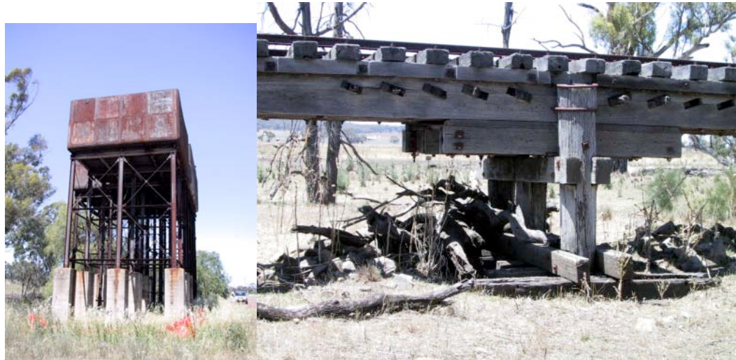
Water supply tank at Merrygoen and some great timber detailing of the railway bridge over the Talbragar River.
