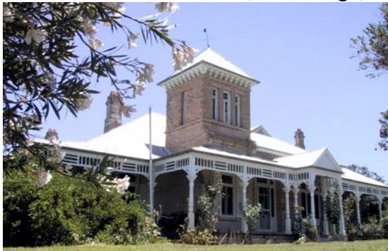
Image of Pine Ridge Station homestead
