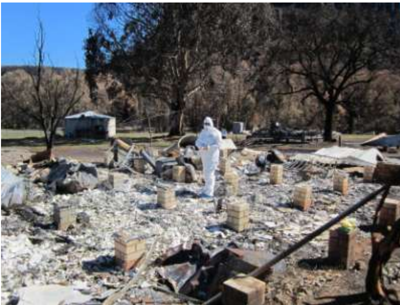
Figure 2 – Burned Down Building within the WSC Local Government Area
