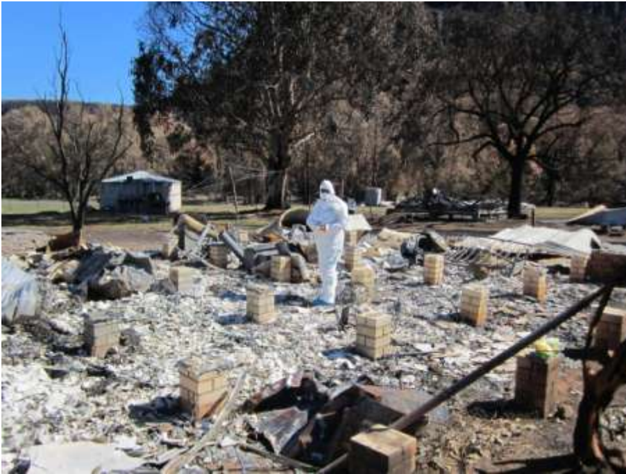
Figure 7 – Example of Fire Damaged Asbestos Cement that is considered friable asbestos.
