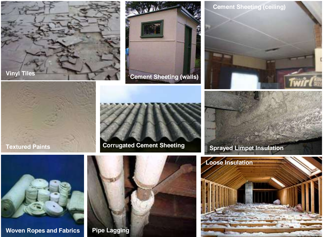
Figure 4 – Typical Asbestos Containing Materials (ACMs) from Bonded Vinyl Tiles to Friable Insulation
