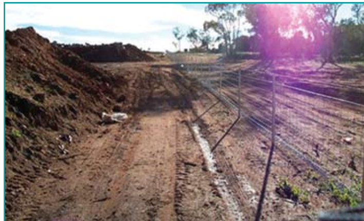
Pig proof fencing with high tensile wires, netting at the base and barbed top wire
