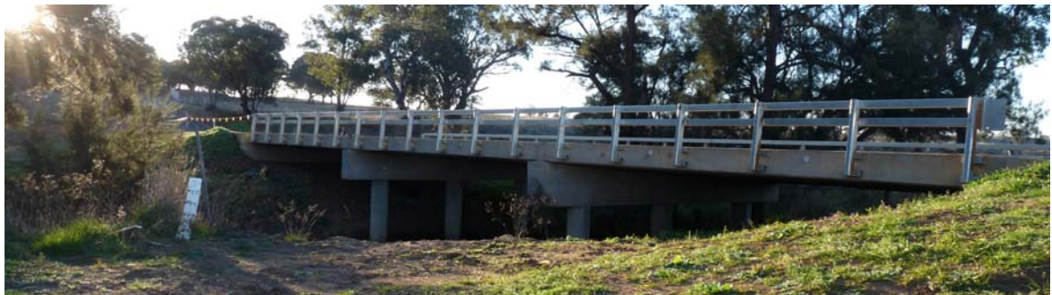
New bridge over Castlereagh River
