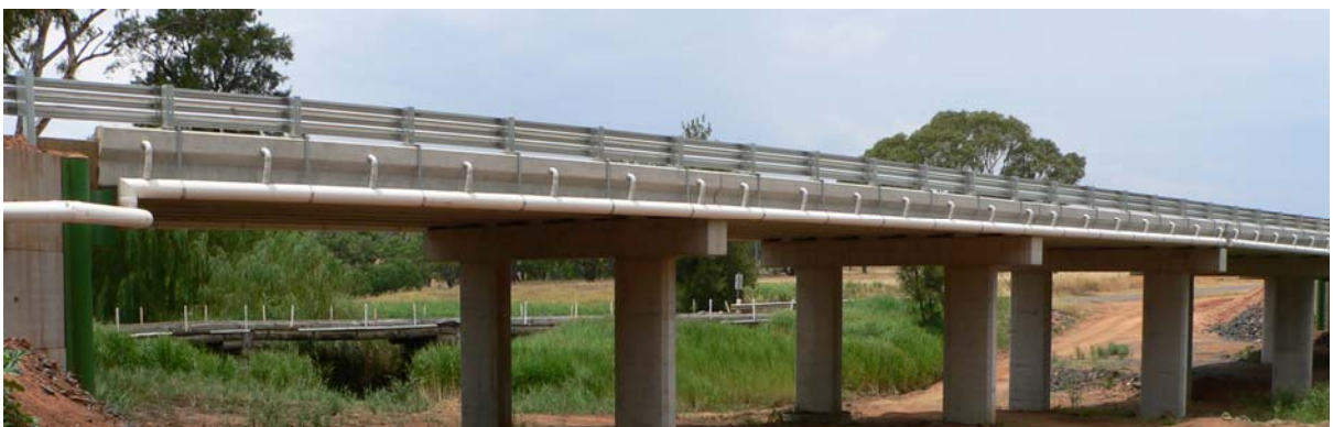
Deringulla Bridge over Castlereagh River
